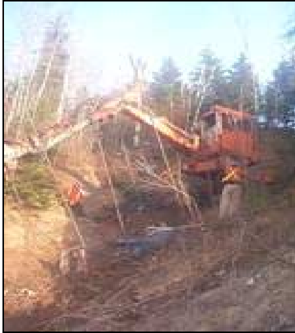
Figure 16: Driving soil nails from slope.
