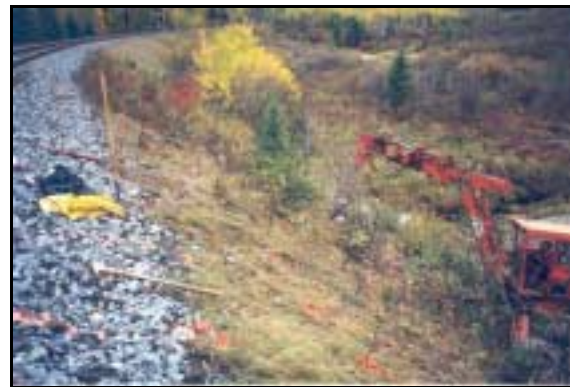
Figure 2: Railway embankment stabilization
