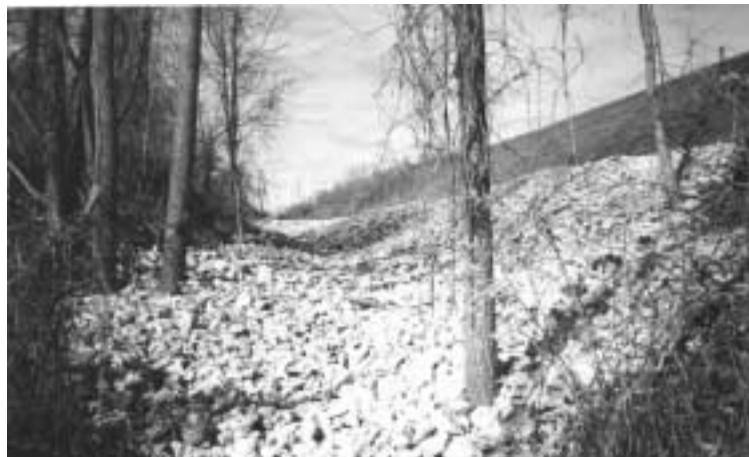
Figure 13 – Completion of embankment stabilization, soil nails and erosion protection installed.
