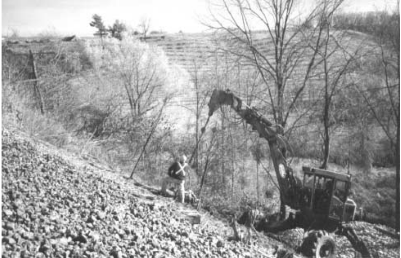
Figure 14 – Installation of soil nails east limit of Site 2 stabilization.
