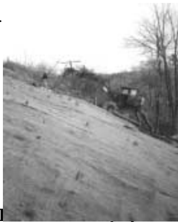
Figure 12 – Site 2, installation of soil nails east limit of stabilization.
